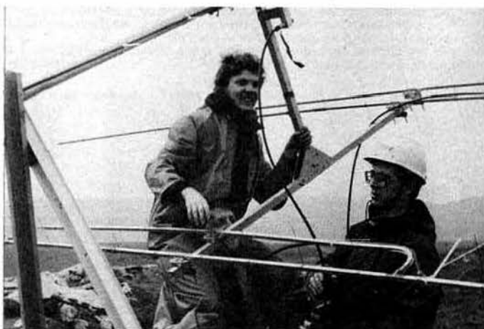
South Manchester RC members G4ROM on G3ZDM, waterproofing connectors on the 432MHz antenna, with G8RGZ giving instructions. Photo: G4MYB
